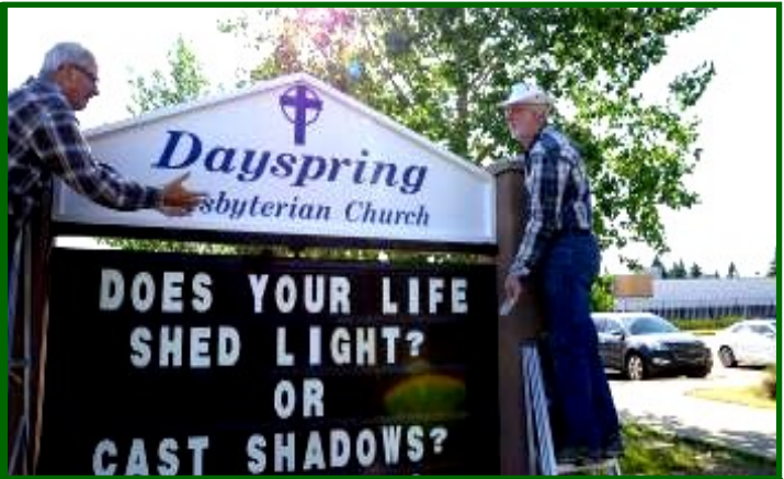
Gary T & John R Complete Repairs on the 40th Ave Sign
